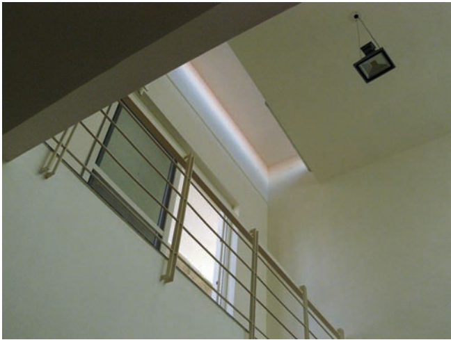
the north light drawn in through a linear stretch of windows facing the north that diffuse the light. This evenly light up the interiors increasing the building efficiency during the day.
