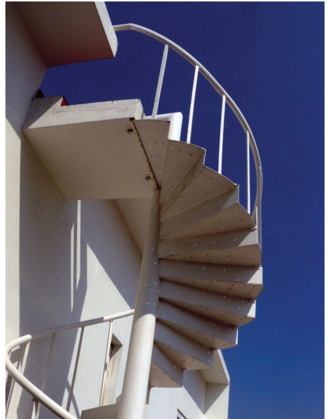
the white spiral steel staircase invokes interest against the horizontality.
